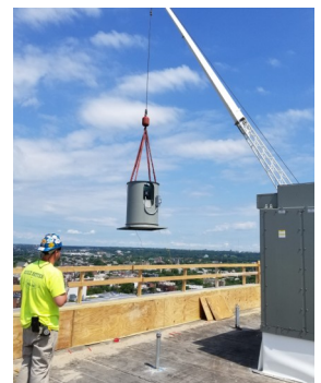
(Pictured clockwise from top to bottom: 3675 Market Street Fans in Place, Mark Koppenhafer signaling the crane, landing the second fan)
