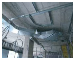
Heat pump system on 3rd floor.
